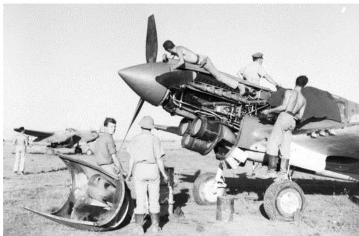
Figure 6. Foggia, Italy. 1943. A Curtiss P40 Kittyhawk fighter bomber of No. 3 Squadron RAAF, having a thorough overhaul.<sup>89</sup>
